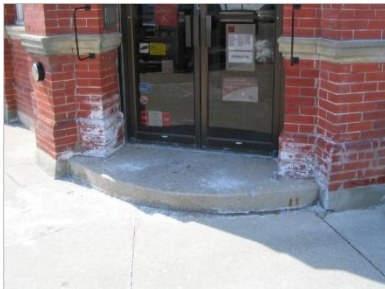
PROTECT FROM SPALLING AT GRADE
