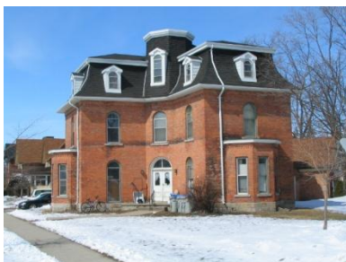
EVIDENCE OF A FORMER FRONT VERANDAH
