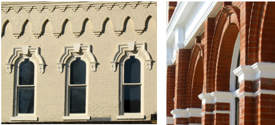
Windows materials and surroundings should be based on those of the original building Goderich, Ontario
