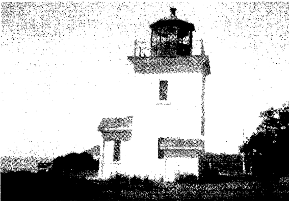
Viewed from the South
